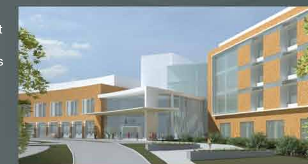
Bergelectric’s proven track record at several UNC venues provides a solid base of knowledge from which to provide exceptional service at the new $200-million Hillsborough campus hospital.
