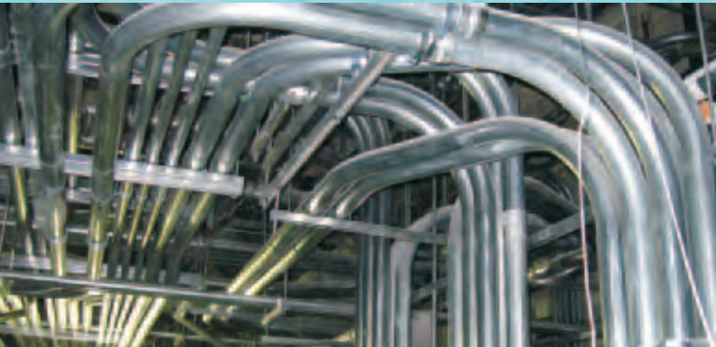
Berg’s 3-D modeling experts are playing a critical role on the state-of-the-art VA Medical Center project—particularly with the volume of overhead feeder conduit installation over three different elevations—through enhanced coordination and potential clash detection with other systems.
